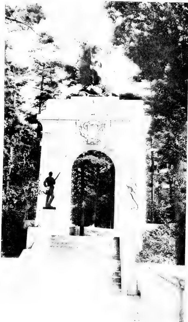
THE ENTRANCE TO ISLAND GROVE
